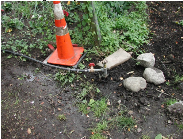
The old irrigation system
